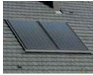
2 vertical collectors mounted in roof integration on mechanical tiles
